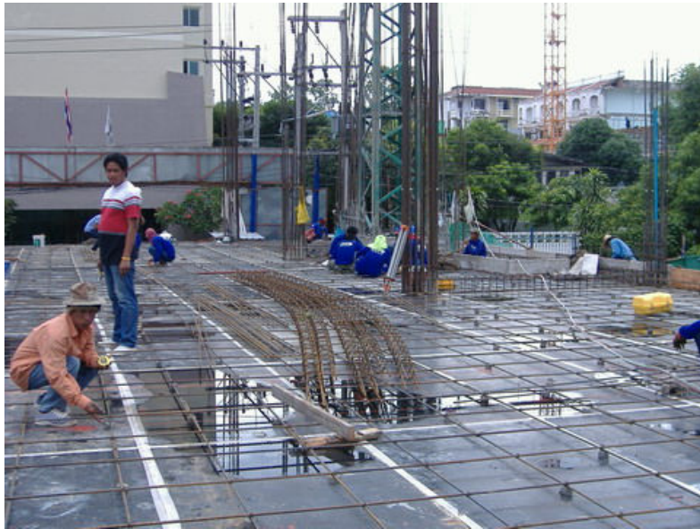
Form Work and Rebar 2 nd Floor
