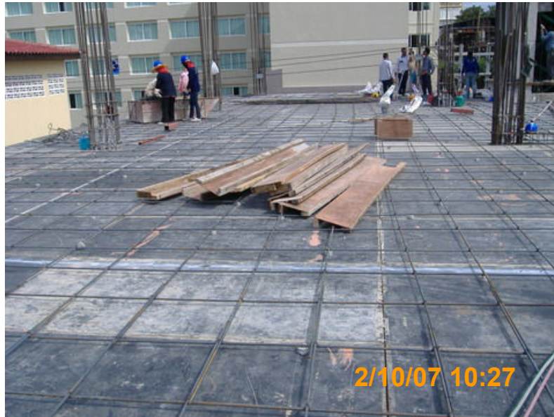
FORM WORK & RE-BAR LEVEL 4 th
