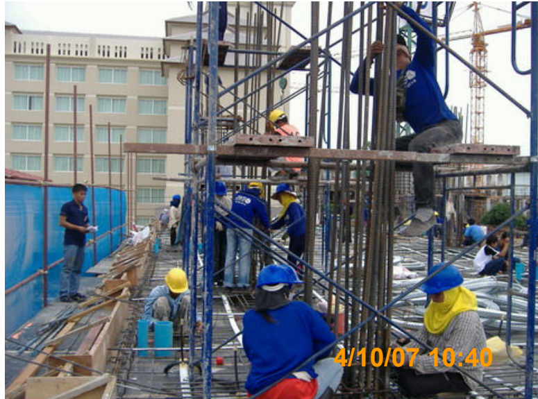
INSTALL RE-BAR LEVEL 4 th TO LEVEL 5 th
