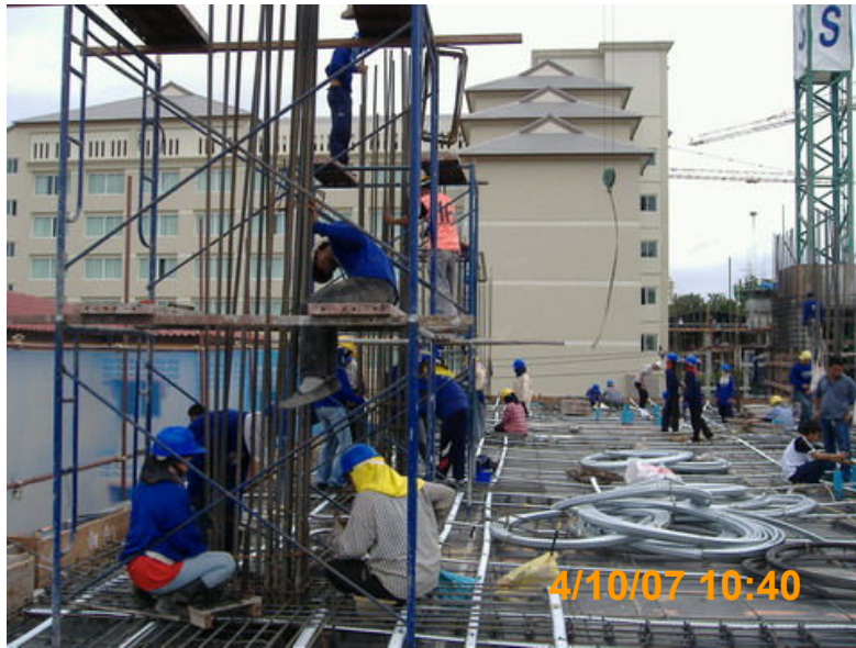
INSTALL RE-BAR LEVEL 4 th TO LEVEL 5 th
