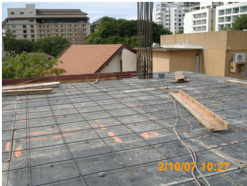
FORM WORK & RE-BAR LEVEL 4 th
