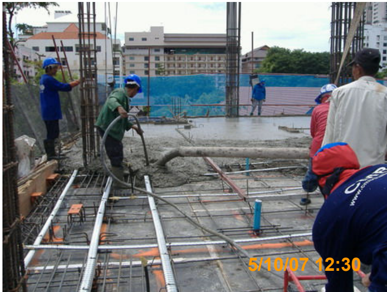
POURING CONCRETE LEVEL 4 th
