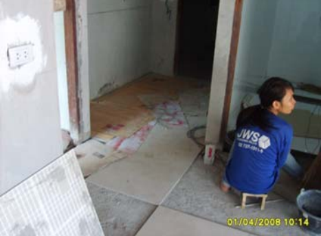
Picture 48: Tiling works at Kitchen Area
