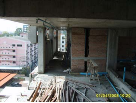
Picture 75: Brick wall and plastering
