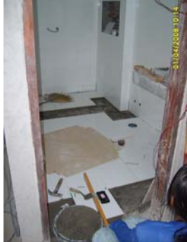
Picture 49: Wall and Floor tiling work in
