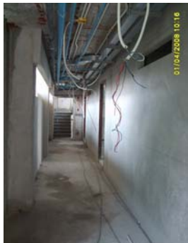
Picture 58: Electricity wire installation at
