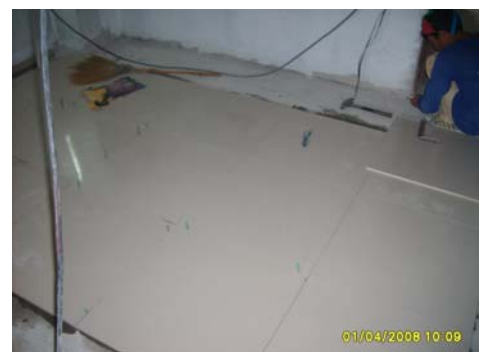
Picture 45: Tiling works at Kitchen Area
