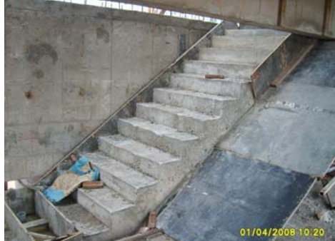
Picture 73: Stair structure to Swimming
