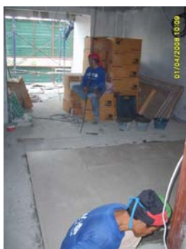
Picture 44: Tiling works at Kitchen Area
