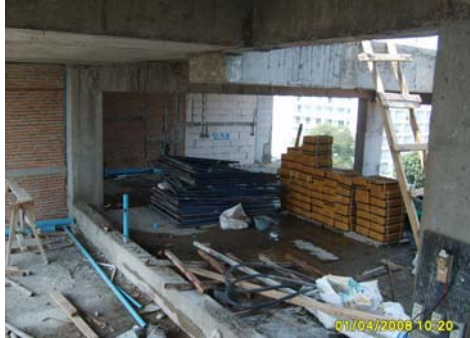
Picture 74: Brick wall and plastering
