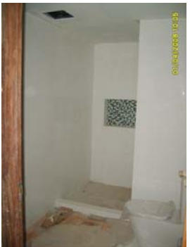
Picture 27: Toilet area
