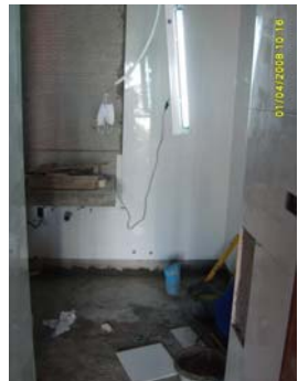
Picture 56: Wall Tiling in Toilet
