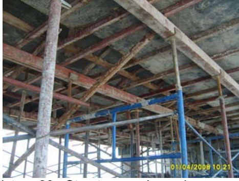
Picture 80: Structure works under
