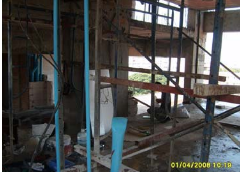
Picture 68: Structure work and
