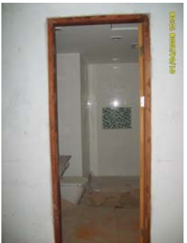
Picture 30: Toilet Area
