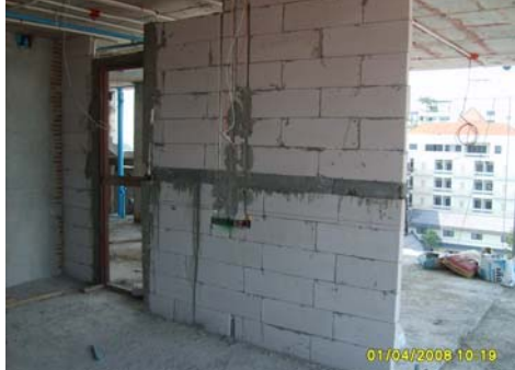
Picture 71: Brick wall works
