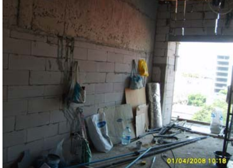
Picture 64: Brick wall and plastering
