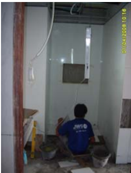
Picture 57: Wall Tiling in Toilet
