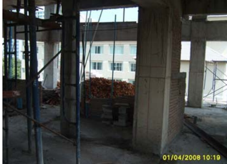
Picture 67: Brick wall and plastering
