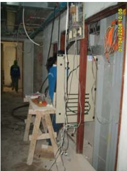
Picture 28: Corridor and Shaft room
