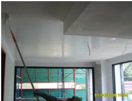
Picture 24: Internal Painting
