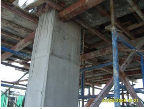
Picture 79: Structure works
