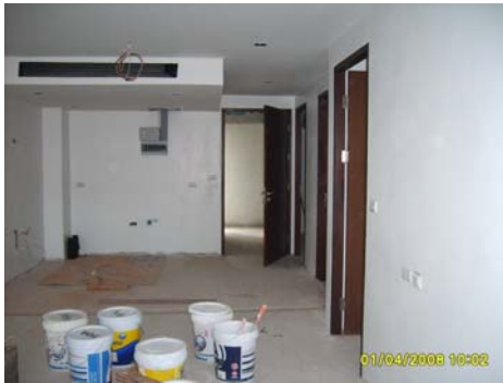
Picture 18: Primary internal painting
