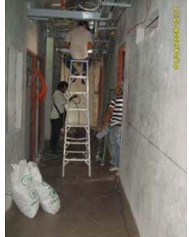
Picture 63: Duck installation at Corridor
