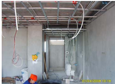
Picture 59: Ceiling frame installation
