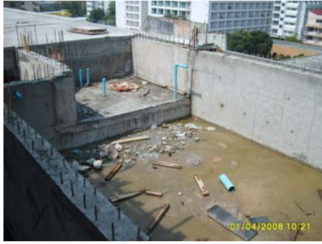
Picture 77: Swimming pool structure works
