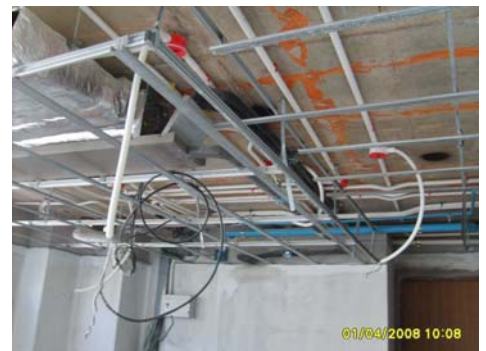
Picture 42: Ceiling works installation
