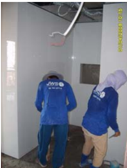
Picture 54: Wall Tiling in Toilet
