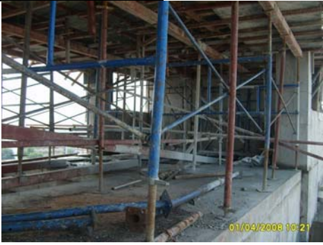
Picture 76: Structure works at Pool deck
