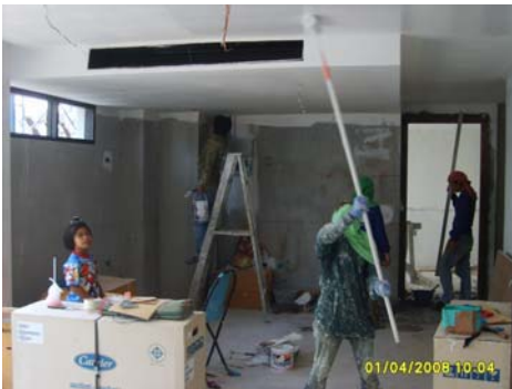
Picture 25: Internal Painting
