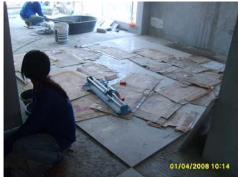
Picture 47: Tiling works at Kitchen Area
