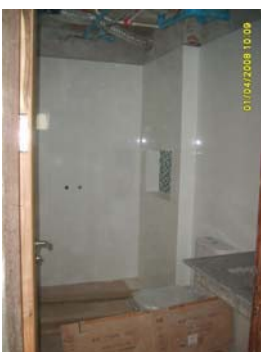
Picture 43: Toilet Tiling and Sanitary ware
