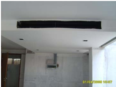
Picture 37: Ceiling block out for Air
