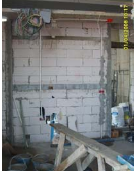
Picture 62: Brick wall and plastering
