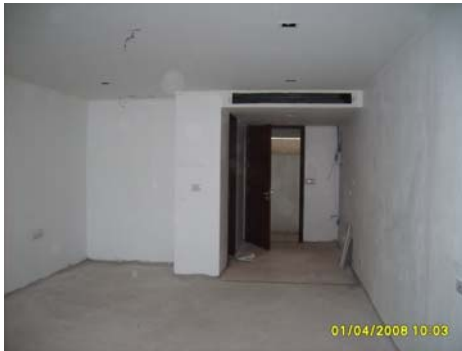
Picture 21: Internal Painting
