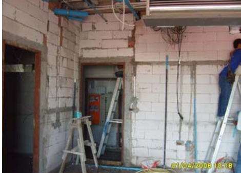
Picture 65: Brick wall and plastering
