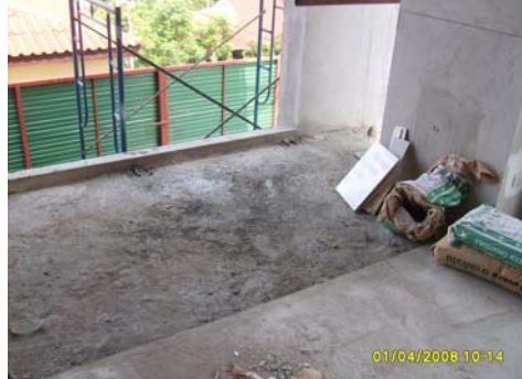
Picture 50: Surface Preparing for Terrace
