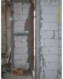
Picture 61: Brick wall and plastering
