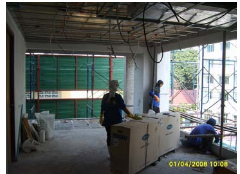
Picture 39: Ceiling frame picture
