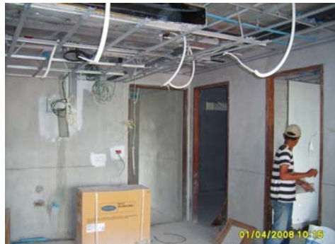
Picture 53: Ceiling frame installation
