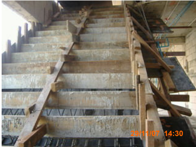
FORM WORK RE-BAR CONCRETE STAIR CASE NO. 1 UP TO 4 th Floor
