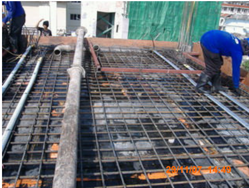
POURING CONCRETE LEVEL 8 th
