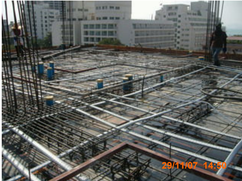
INSTALL RE-BAR & POST-TENSION LEVEL 8 th
