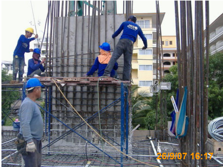
Re-Bar for Lift Level 3 rd
