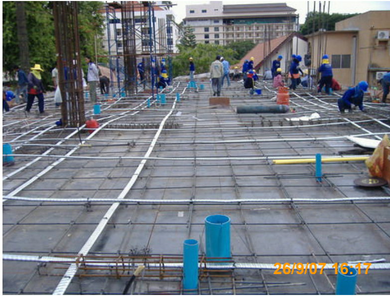
Block Out and Sleeve Level 3 rd
