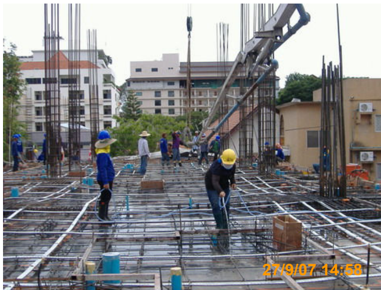
Re-Bar & Post-Tension Level 3 rd
