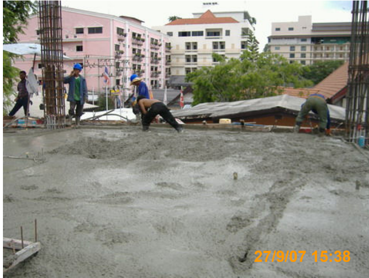
Concrete Slab Level 3 rd
