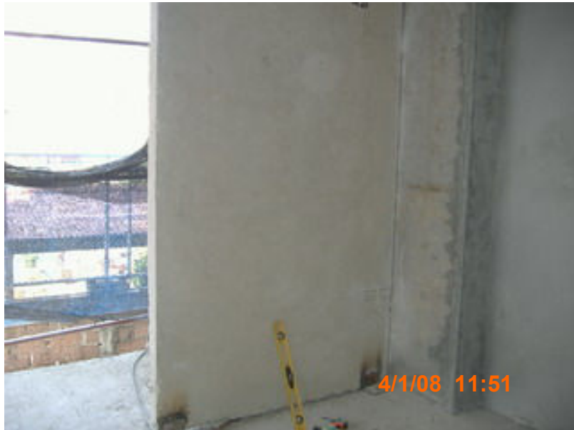
INSTALL PRECAST WALL
