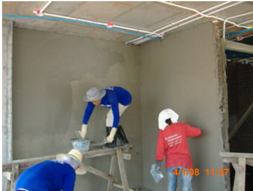
PLASTERING WALL LEVEL 2 nd & INSTALL CONDUIT
